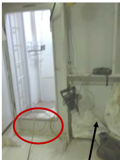
Figure 3. 12" H door threshold creates a tripping hazard; hatch threshold is ~4" H and is ~24" x 29"
